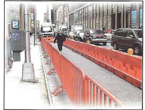
Temporary Pedestrian Walkway
